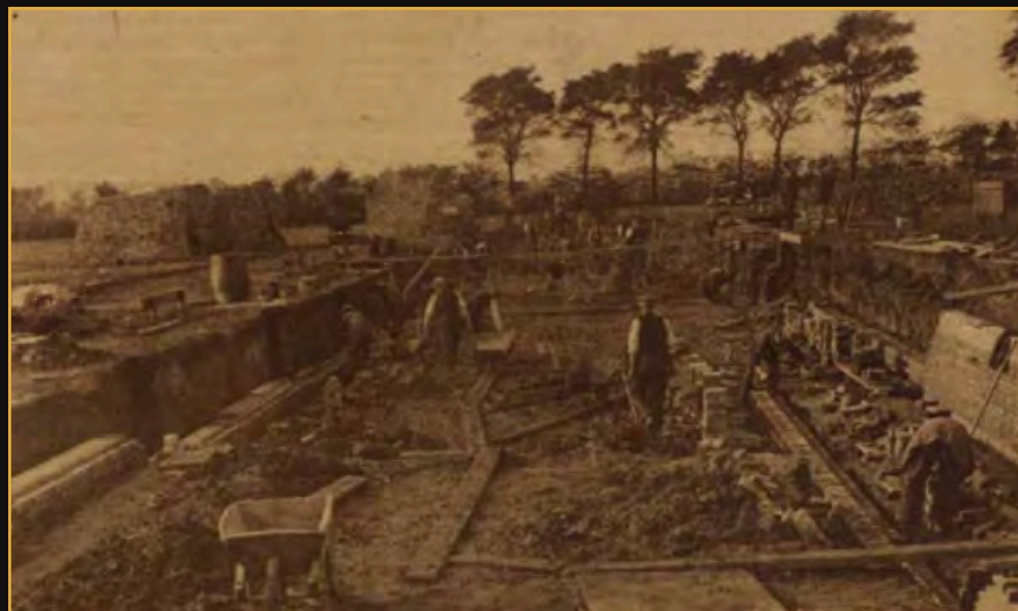
Digging the Foundations of Westcliff High School for Boys, 1924
